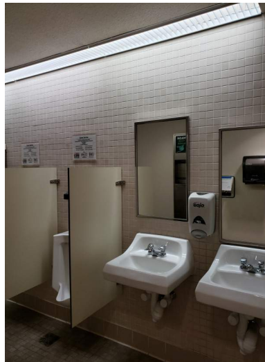
Room 1001, typical restroom.
