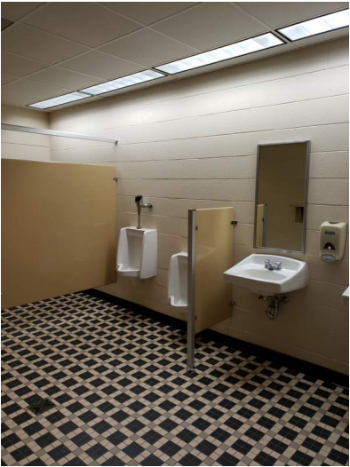
Room 313, typical restroom.
