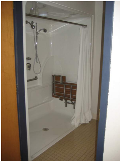
Typical dressing room shower.
