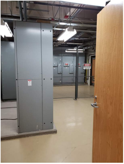
Room 203, looking east.
