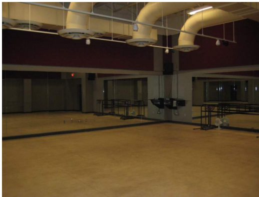
Room 101D, looking east.
