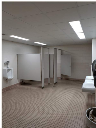
Room 1002, looking north.
