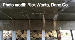
Rusting and concrete damage caused by corrosion from chlorides
