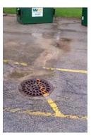
Sediment in stormwater runoff being carried into storm drain on UWGB campus
