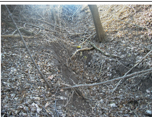
Photo 3.7.4: Looking towards 24" Weidner Center Outfall
