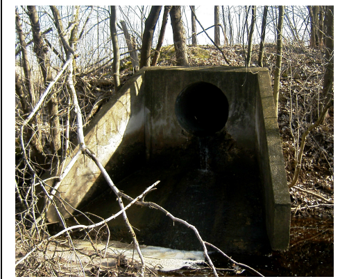
Photo 3.7.2: 36" Mahon Creek Outfall
