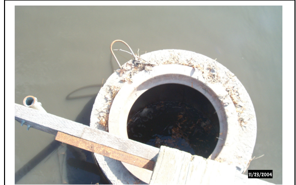
Photo 4.3.2: Golf Course Outlet Structure
