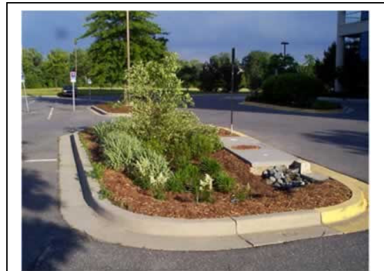
Photo 7.0.4: Parking Lot Biofiltration Area
