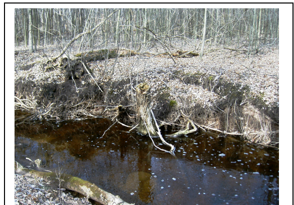
Photo 3.9.2: Mahon creek Bank Erosion
