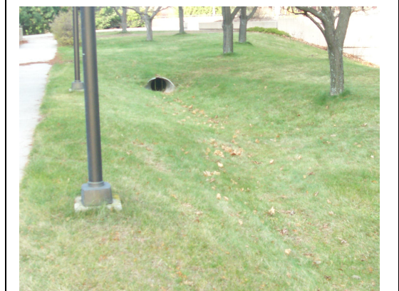
Photo 7.0.7: Swale on UWGB Campus
