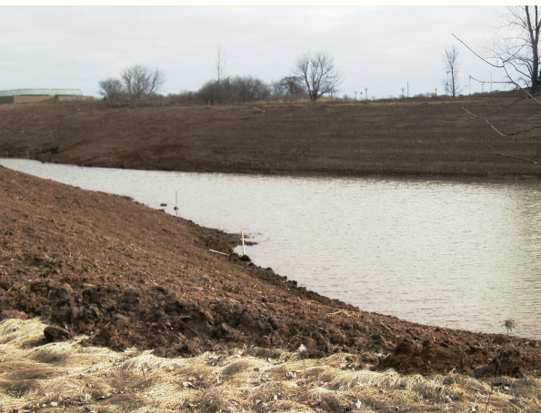
Photo 4.3.3: Phoenix Sports Center Wet Pond
