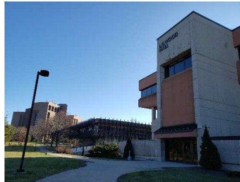
(2) Wood Hall/Rose Hall/Cofrin Library, looking east down Main Entrance Drive. No clear points of entry or visitor parking along entrance.
