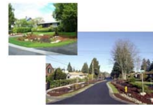
Figure 2. Rain Gardens in Seattle, WA. (Low Impact Development Center, Inc. 2004).
