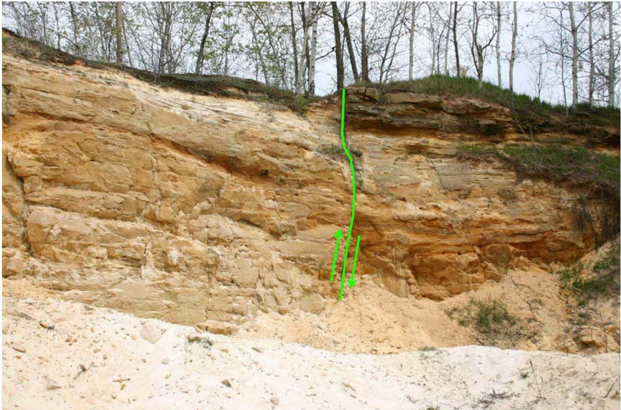
Figure 2. Exposure of the St. Peter Sandstone near Seymour, Wisconsin illustrating heavily fractured sandstone and a dip-slip fault with about 3 feet (1 m) of vertical offset (right hand side is downthrown).
