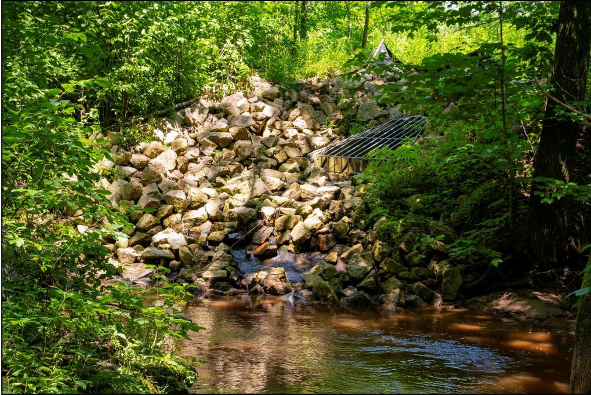
**Figure C33.** Rock drainage field designed to dissipate high energy water flow from culvert along Mahon Creek.
