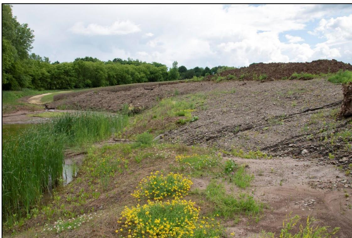
**Figure C16.** Brown County Public Works Project along Lake Largo Road in the Mahon Creek watershed (2020). Although measures were implemented to reduce surface runoff of water and sediments, stream and riparian habitats have been altered significantly.
