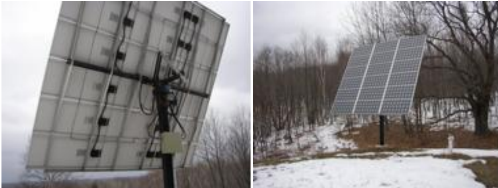
Back and front side of a single axis tracker, which follows the sun's apparent movement east to west daily.
