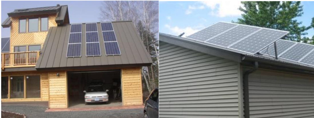
Example. On the left, a 1.9 kW roof mounted array on a standing metal seam roof. On the right, a 2.94 kW system on a corrugated metal roof
