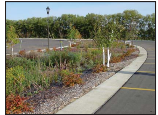
Parking Lot Buffer Strips These can be an aesthetic enhancement to any parking lot. Buffer strips can be constructed with curb and gutter, which often contain stone rip rap strips where curb cuts are located to slow the velocity of water into the area. Others are constructed with an at-grade curb strip, as depicted above. Photo courtesy of the Minnesota Erosion Control Association, www.mnerosion.org/meca_lid_mnpls.htm
