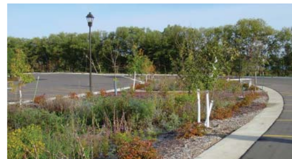
The Minnesota Landscape Arboretum This example demonstrates that pedestrian walkways can accommodate foot traffic at designated locations that transect the buffer strips. Photo courtesy of the Minnesota Erosion Control Association, www.mnerosion.org/meca_lid_mnpls.htm
