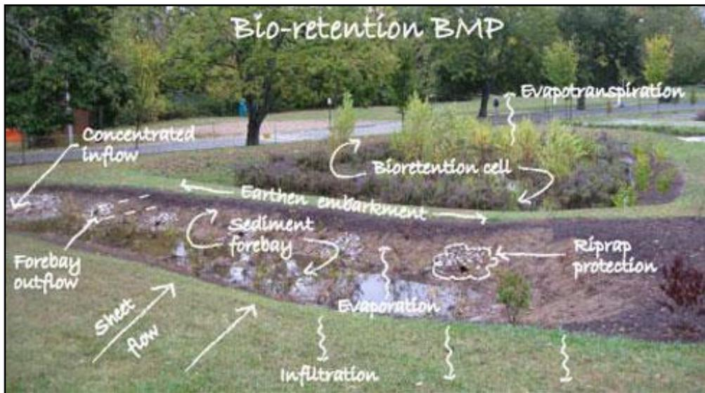
**Figure 3.4: Bioretention cell and forebay designed to receive runoff from a nearby parking lot (Virginia Tech University)**
