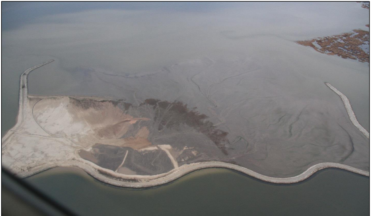
Photograph of the Cat Island Wave Barrier facing southwest, featuring the westernmost cell, which has been filled with sandy dredge material within the last few years. Photograph taken by Erin Giese on 2 December 2016.
