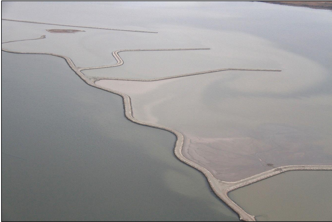
Photograph of the Cat Island Wave Barrier facing southwest, featuring the middle “cell,” which was recently filled with dredge material and historic Cat Island in the upper left. Photograph taken by Erin Giese on 2 December 2016.
